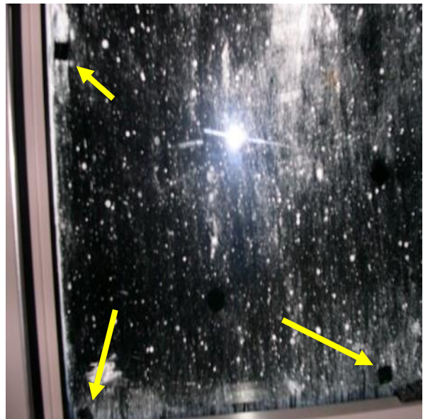
Photo Above shows an installed window with heavy condensation on Glass. Different patterns are visible within the condensation including the outline of separator pad marks on glass. As above there are no visible marks present on this glass in the absence of condensation.
